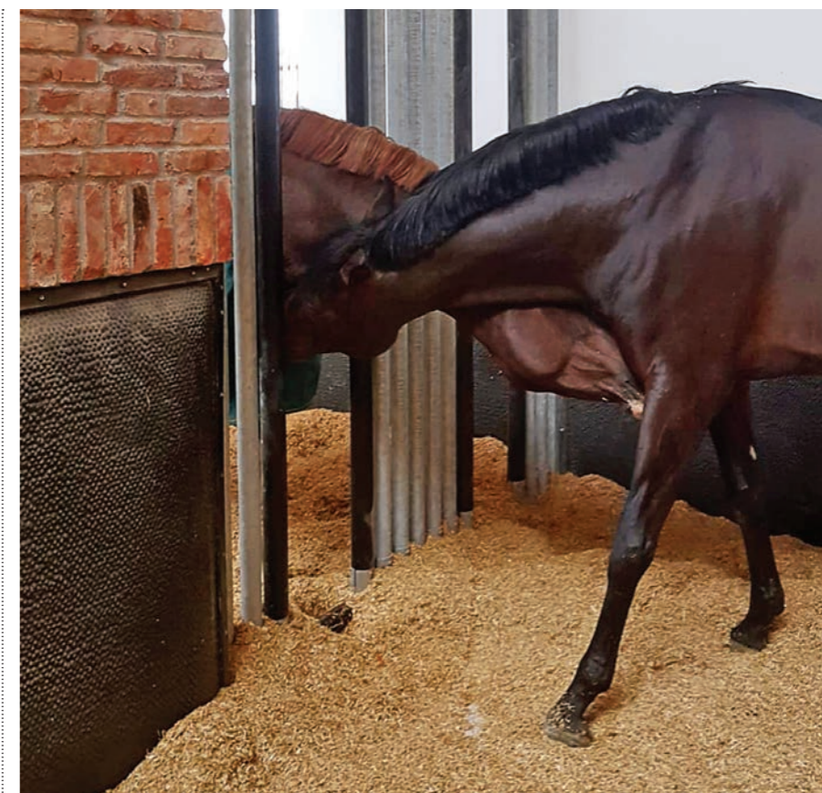
ABOVE: In some European yards, a progressive stabling concept incorporates grids between boxes permitting restricted tactile contact.
